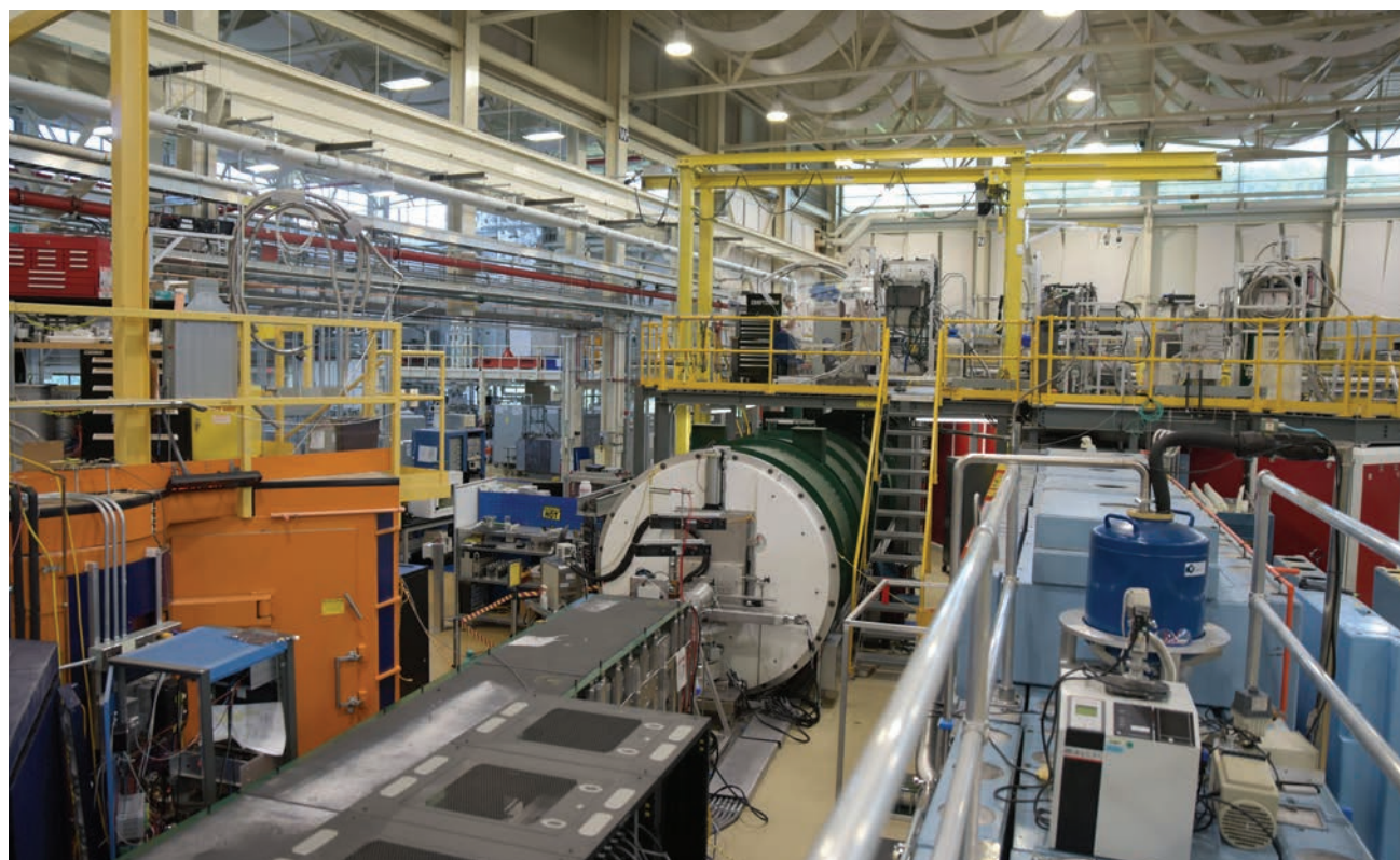
▲ A view of the guide hall at the NIST Center for Neutron Research, which is ramping up after a shutdown of five-plus years that was triggered by a refueling incident. The black infrastructure and the large cylinder are parts of the Very Small Angle Neutron Scattering instrument. To its right is a beamline feeding another instrument, the Disk Chopper Spectrometer. The orange machine at left is part of the High Flux Backscattering Spectrometer. (Photo by Rich Press/NIST.)
