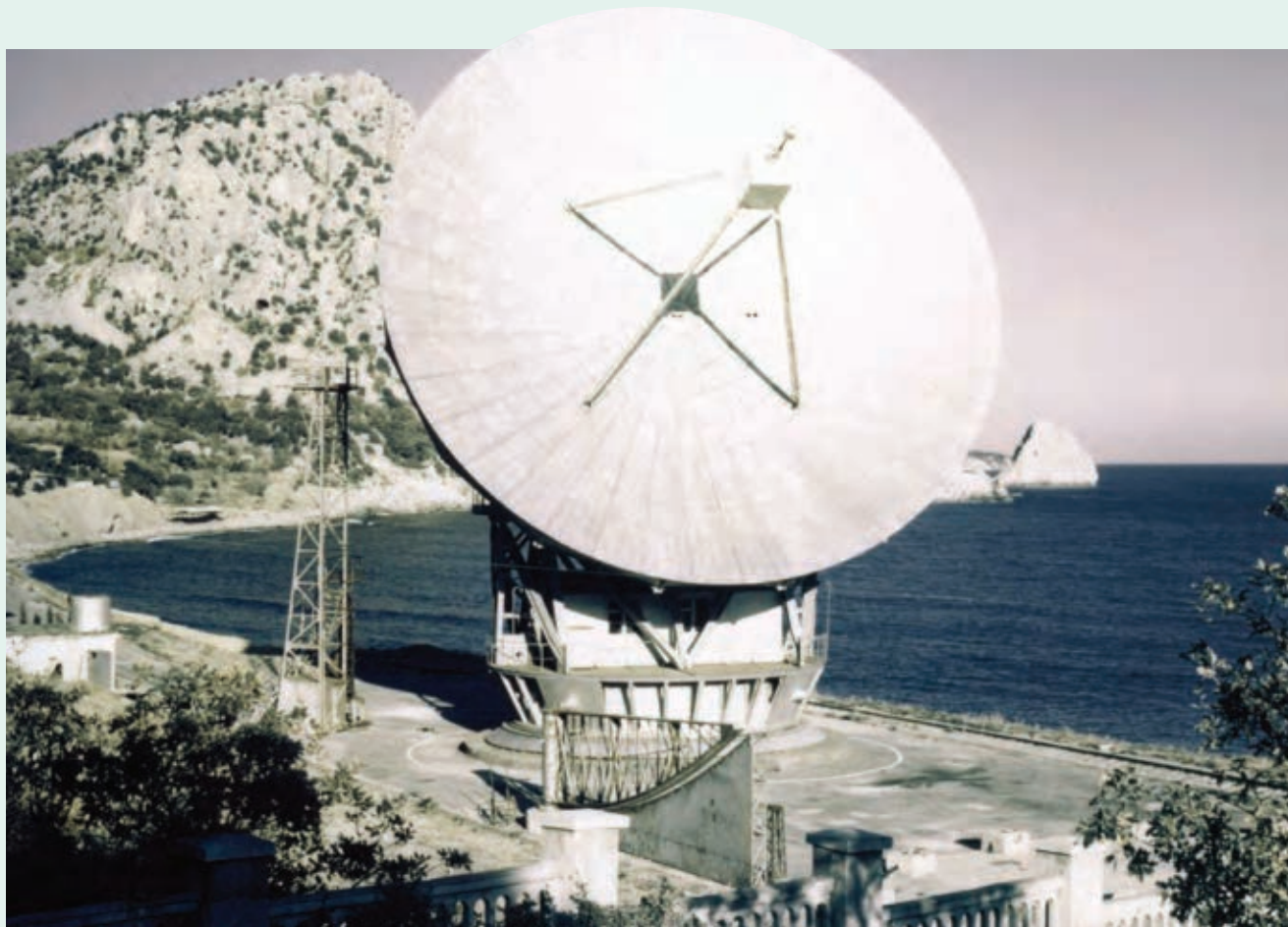
THE 22-METER RADIO TELESCOPE at the Simeiz Observatory in Crimea used in the 1969 US–USSR VLBI experiment. (Photo by K. Kellermann, courtesy of NRAO/AUI/NSF/CC BY 4.0.)
