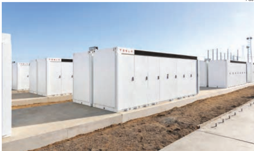
TESLA MEGAPACK lithium-ion batteries located at a PG&E substation in Northern California. When completed later this year, the facility will be capable of dispatching energy to the grid at the rate of 182 MW for up to four hours.
