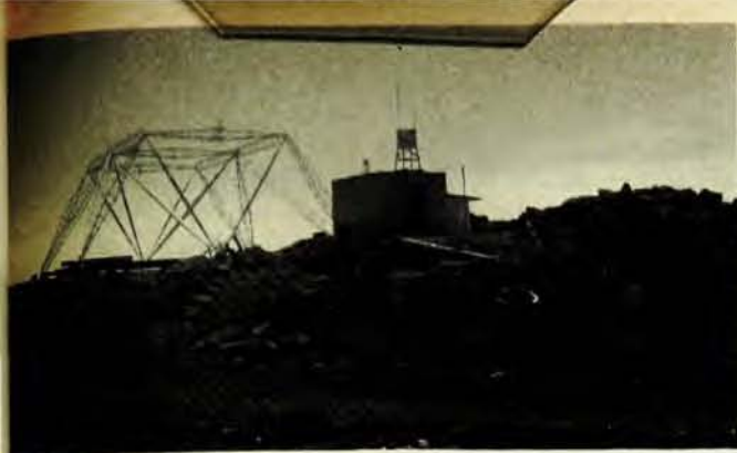
Directional antenna system on summit (10 025 feet) of Mt. Haleakala, Island of Maui. Building at right of antenna houses receivers and other equipment. Antenna system can be rotated about vertical axis passing through center of structure. Antenna forms receiving unit of a Lloyd's mirror arrangement, using reflecting surface of the ocean below, and permitting good resolution for radioastronomy studies of radiation received from stars and other sources in the galaxy. Built by Grote Reber, with cooperation of Hawaiian Telephone Co. and University.
