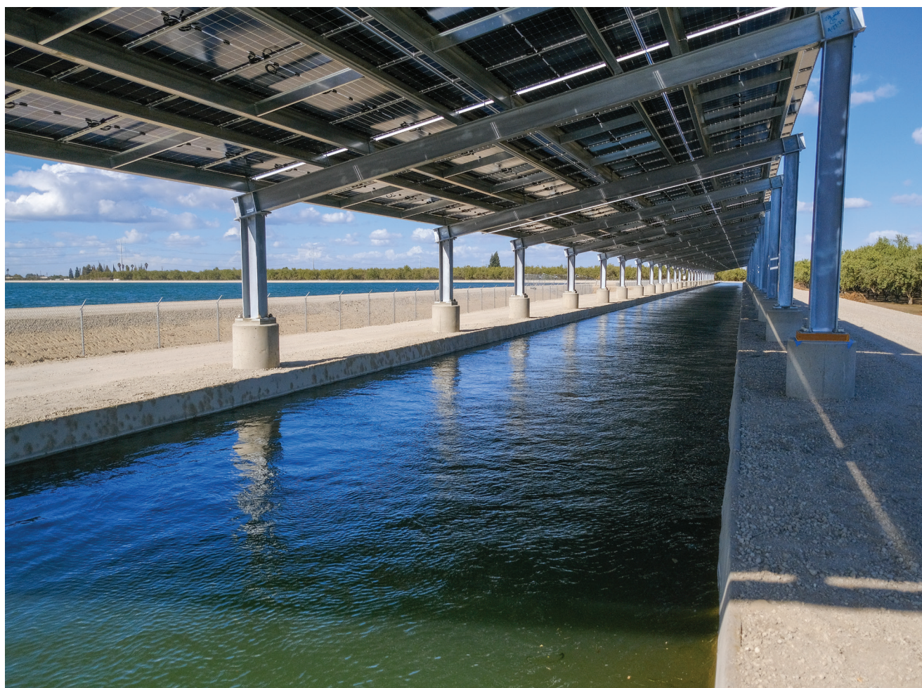
SOLAR PANELS shade a Turlock Irrigation District canal in Stanislaus County, California. Researchers studying pilot projects in California and Arizona are quantifying the advantages and disadvantages for water and land conservation. (Photo courtesy of Turlock Irrigation District.)
