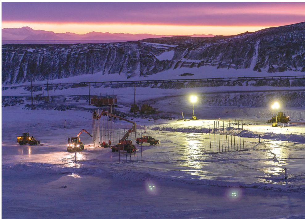
CREWS AT MCMURDO STATION in Antarctica work in 2015 to repair cracks in a pier. NSF had planned to allot some of the $60 million it requested for Antarctic infrastructure upgrades in fiscal year 2025 to replacing the pier, which is used to receive shipments of supplies. (Photo by Bill Henriksen/USAP/NSF/CC BY-NC-ND 4.0.)
