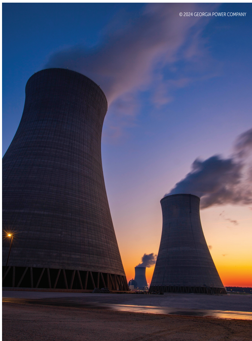
COOLING TOWERS at the Vogtle plant in Georgia, where two new reactors went on line in the past year. The plant hosts 4 of the now 94 operating reactors in the US. The reactors' huge time and cost overruns exemplify challenges facing the expansion of nuclear capacity.
