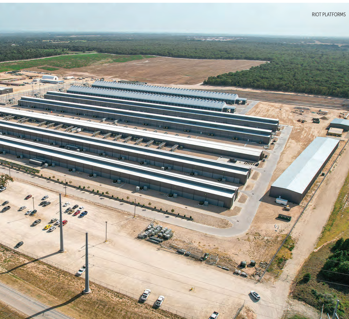
RIOT PLATFORMS'S bitcoin mining facility in Rockdale, Texas. With an installed capacity of 700 MW, it is the largest bitcoin mining farm in North America. The company, which produced 6626 bitcoins in 2023, is constructing a larger farm in the state that will have a capacity of 1 GW.
