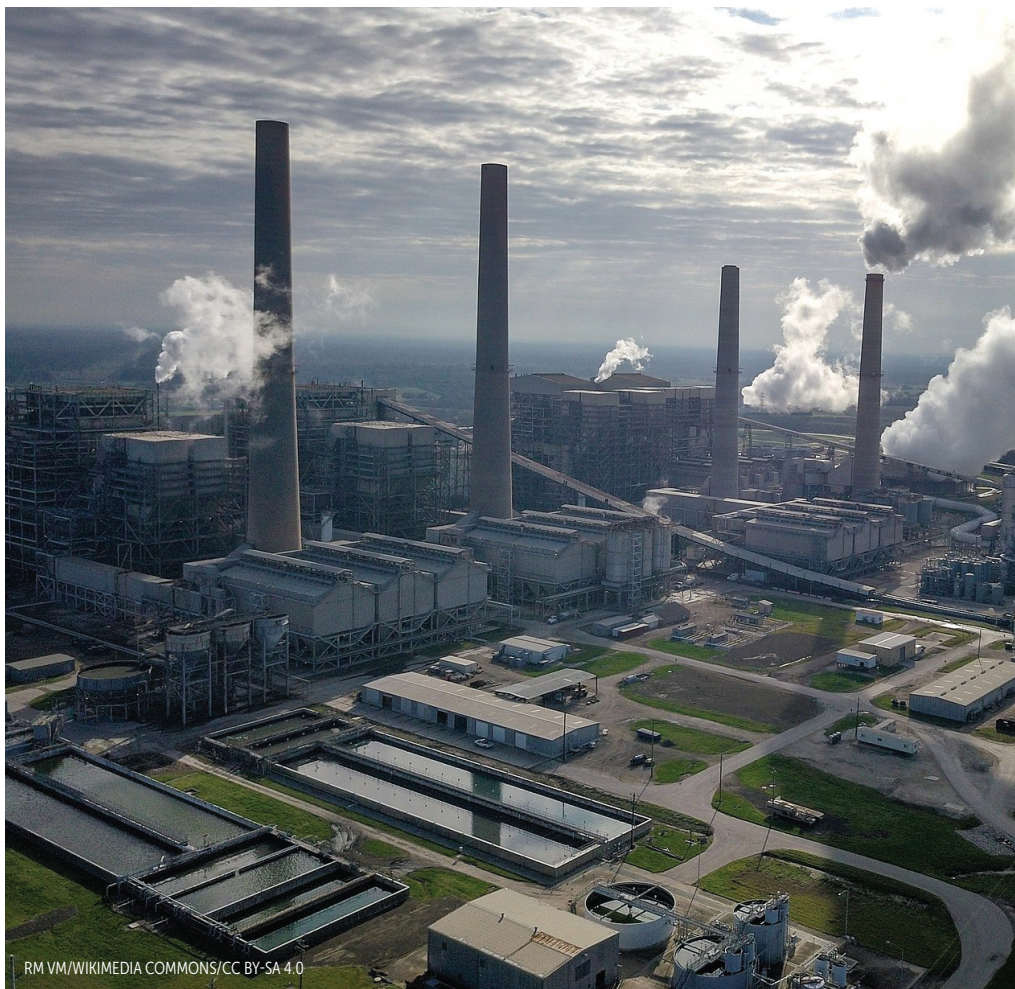
THE PETRA NOVA plant in Thompsons, Texas, was the only US power plant to successfully capture carbon dioxide from postcombustion at a commercial scale. The CO 2 was compressed and piped to an oil field for enhanced oil recovery. The system operated from 2017 until 2020, when low oil prices made capture uneconomic.
