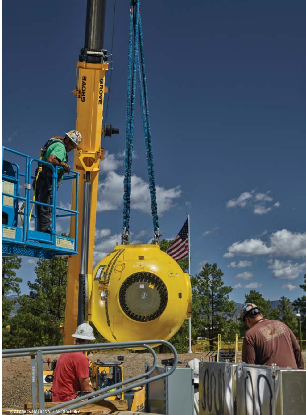
A BLAST CONTAINMENT chamber is lowered into place at the Dual-Axis Radiographic Hydrodynamic Test facility at Los Alamos National Laboratory. Explosive tests on mock pits made from surrogate metals are used to help determine how plutonium will compress as the pit of a nuclear weapon implodes.
