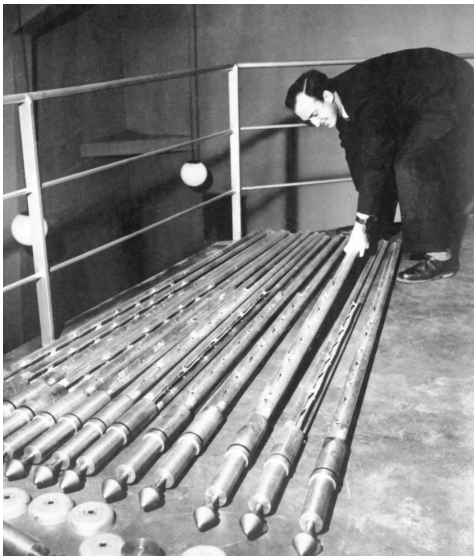
FIGURE 2. RODS OF URANIUM FUEL for the Joint Establishment Experimental Pile reactor, pictured in 1951. (Courtesy of the Norwegian Museum of Science and Technology, CC BY-SA 4.0.)
