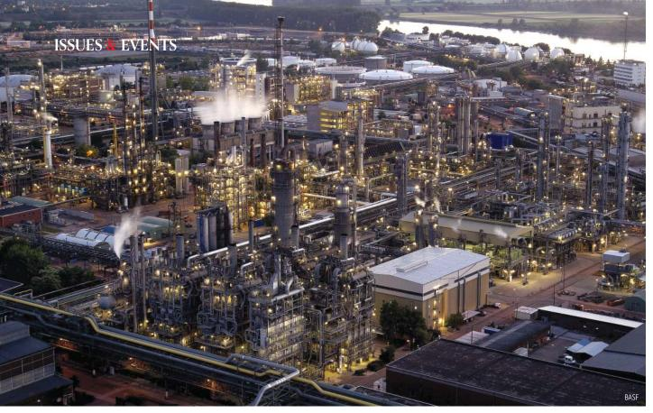
**STEAM CRACKERS**, such as the ones in this BASF facility in Ludwigshafen am Rhein, Germany, require a significant amount of fossil energy to break down long-chain hydrocarbons into smaller, more usable products. The reactions are typically conducted at about 850 °C. Crackers are one of the largest sources of  $CO_2$  emissions in the manufacture of petrochemicals.
