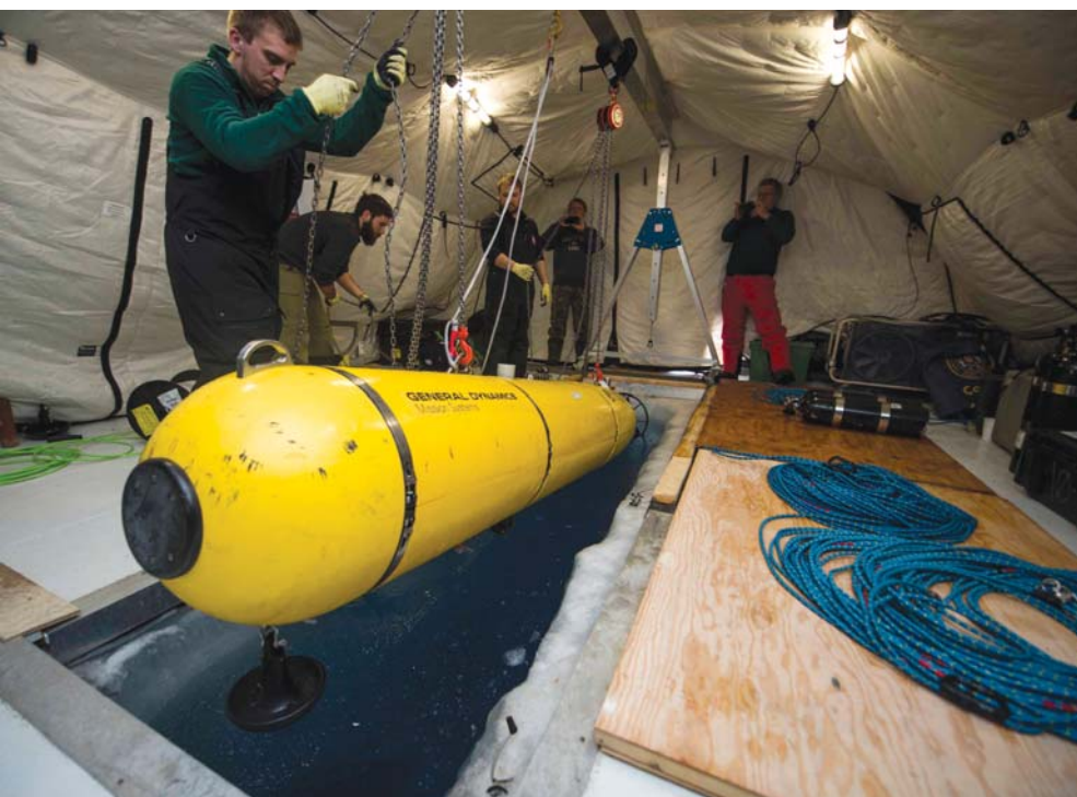
SCIENTISTS FROM MIT lower a sound array through a hole in the ice at the navy ice camp in March 2018. (Courtesy of the Arctic Submarine Laboratory.)
