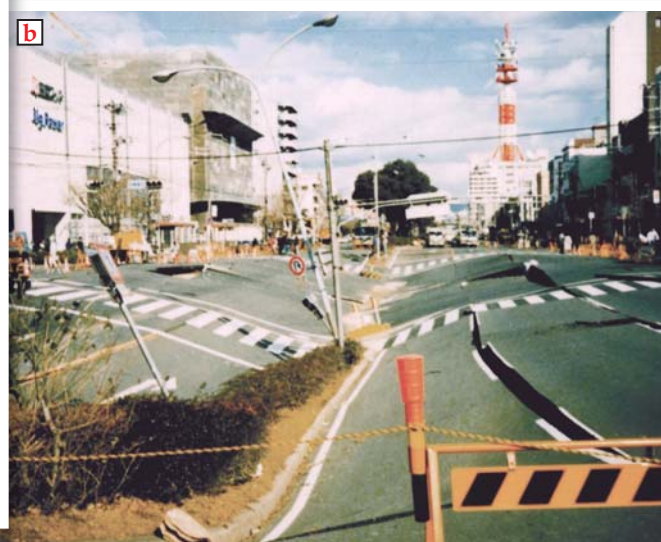
FIGURE 3. THE UNDERGROUND DAIKAI STATION in Kobe, Japan, collapsed during a 1995 earthquake. (a) The reinforced concrete columns supporting the roof gave way and (b) the street above the station sank in a 100 m × 20 m area; in some places, it fell as much as 2.5 m. The failure disproves the myth that underground structures are safe against earthquakes. (Photographs courtesy of Shunsuke Sakurai, Kobe University.)
