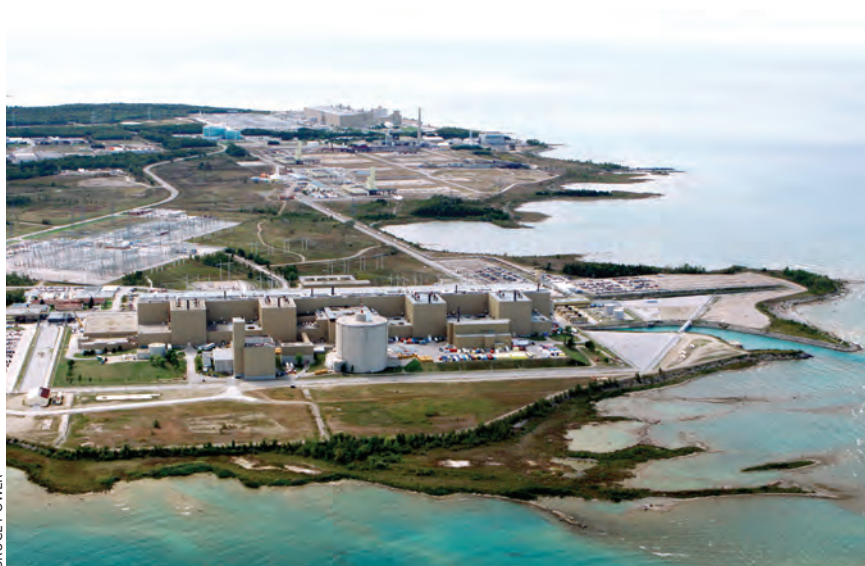
THE BRUCE NUCLEAR GENERATING STATION on Lake Huron is the largest nuclear power plant in North America. Its eight CANDU reactors produce 30% of Ontario's electricity. Four of the reactors are in the foreground; the others are visible in the background.
