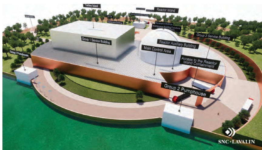
A RENDERING OF A SMALL MODULAR REACTOR design from SNC-Lavalin. The heavy-water-moderated reactor would produce 300 MW of electricity.
