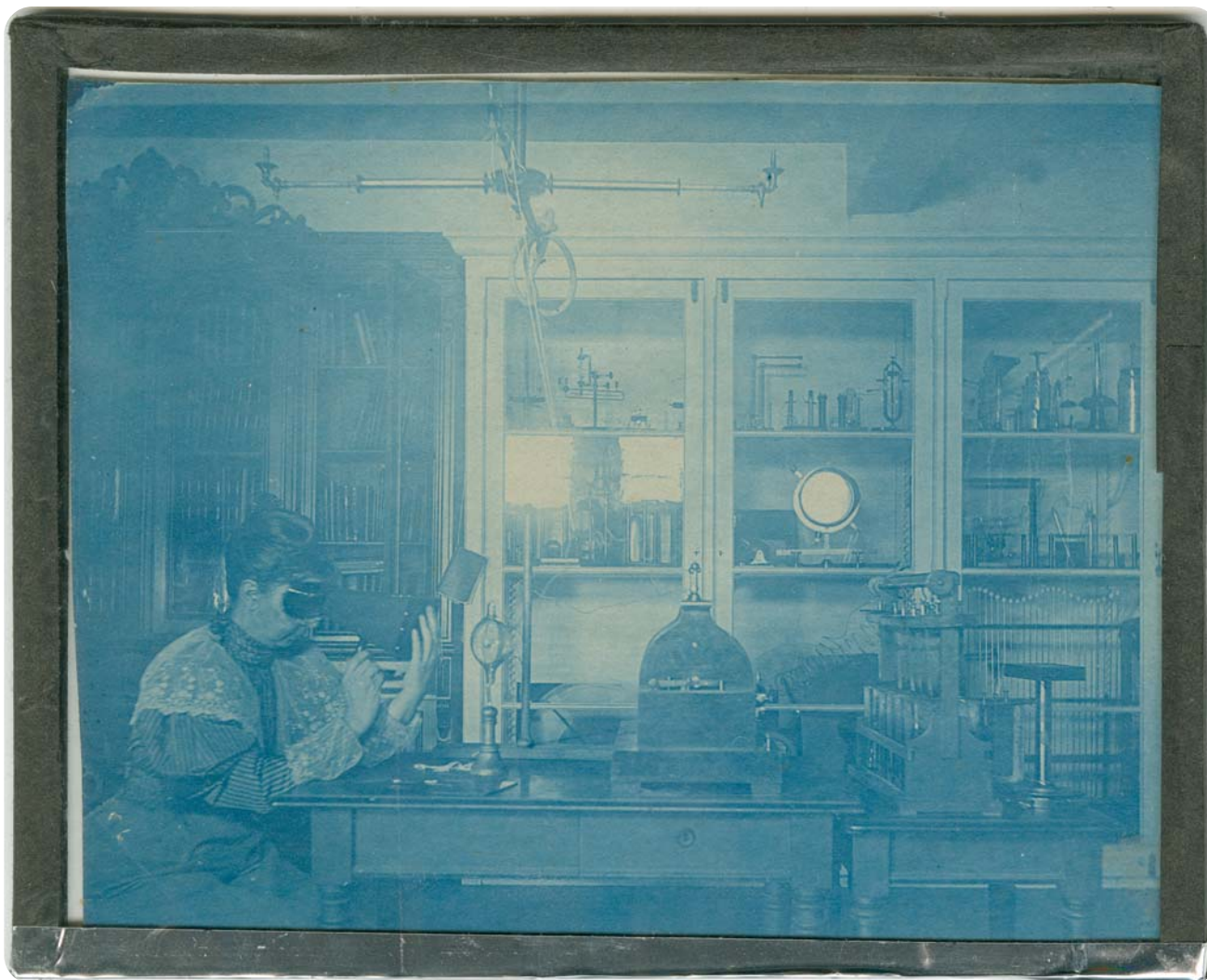
FIGURE 1. SARAH FRANCES WHITING (1847–1927) USING A FLUOROSCOPE to examine the bones in her hand in Wellesley College's physics laboratory, circa 1896. On the table in front of her is a Crookes tube mounted on a stand and an induction coil to modulate the voltage. (Courtesy of Wellesley College.)
