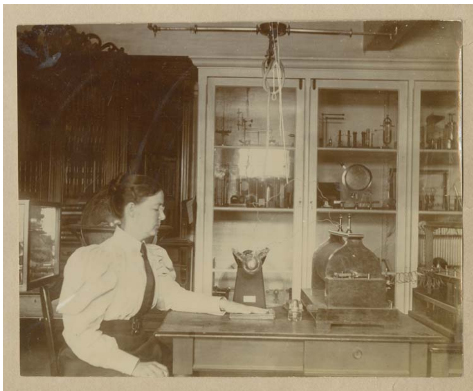
FIGURE 3. SARAH FRANCES WHITING'S COLLEAGUE MABEL CHASE PLACES HER HAND ON A GLASS PHOTOGRAPHIC PLATE , below a Crookes tube, to take a radiograph of the bones of her hand in Wellesley's physics laboratory, circa 1896. (Courtesy of Wellesley College Archives, Library & Technology Services.)
