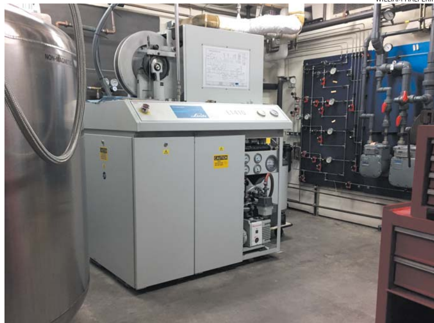
THE CENTRAL HELIUM FACILITY at Northwestern University can liquefy up to 50 liters per day from instruments across the campus.
