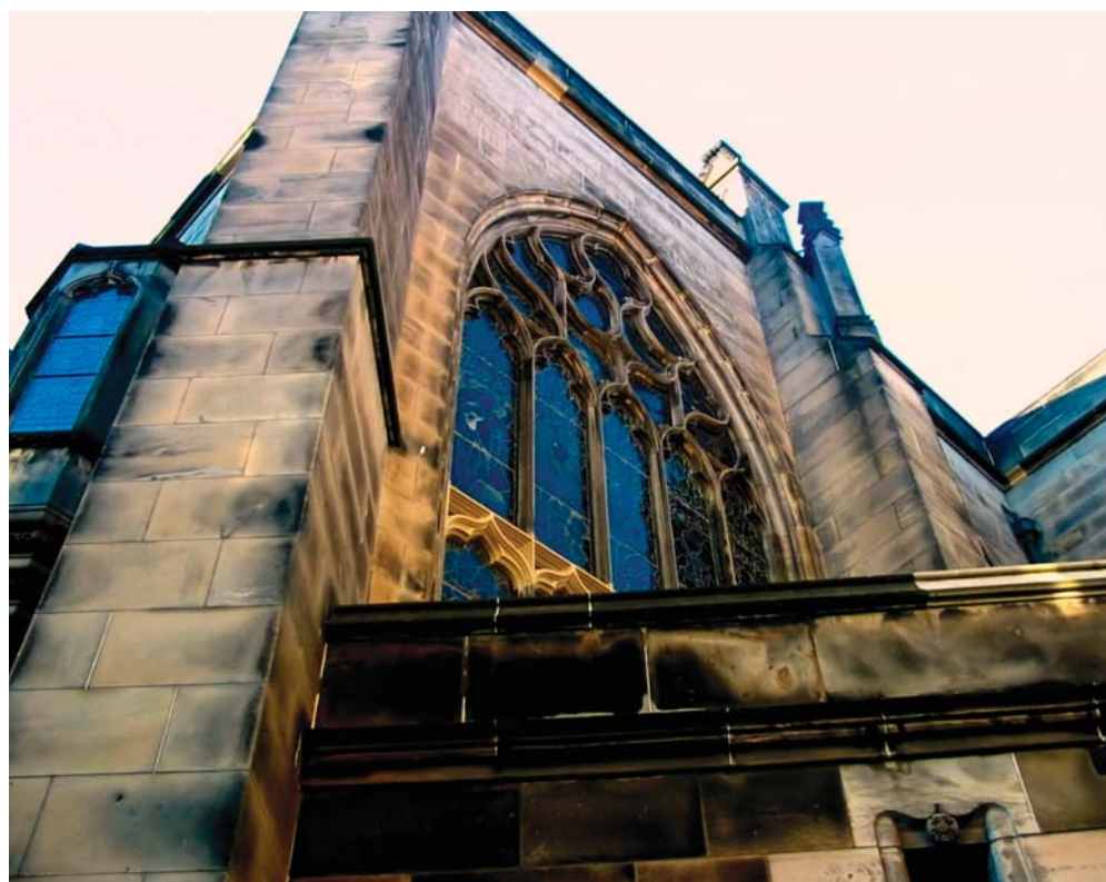
FIGURE 1. ST GILES' CATHEDRAL IN EDINBURGH. Unregulated coal burning from the Industrial Revolution up to the 1950s led to many soot-blackened buildings in the UK. (Photograph by Rachele Burnside/Shutterstock.com.)
