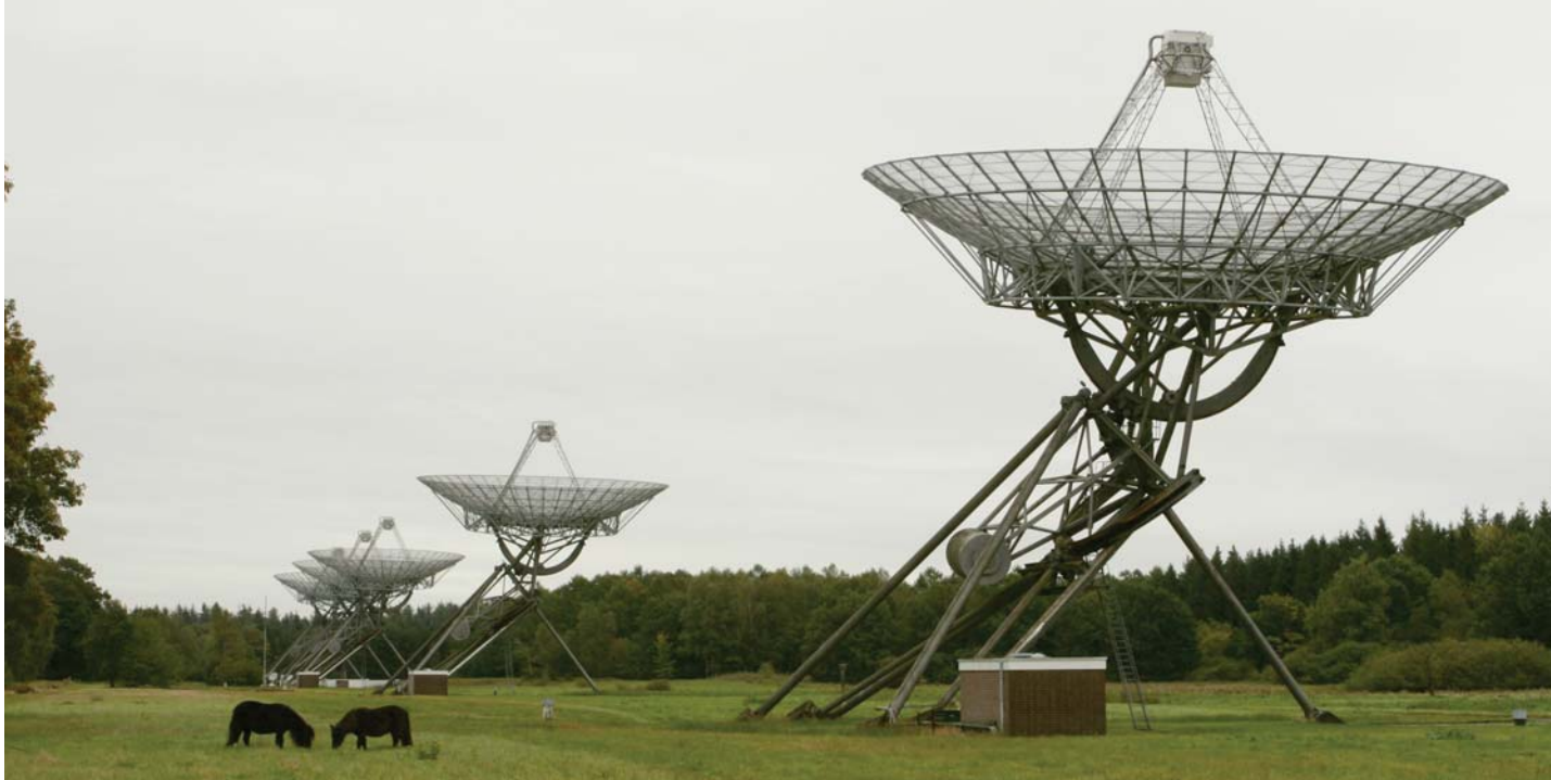
THE WESTERBORK SYNTHESIS RADIO TELESCOPE in the Netherlands brings 14 dishes, each 25 m in diameter, to the European Pulsar Timing Array project. Together, they have an effective diameter of 94 m.
