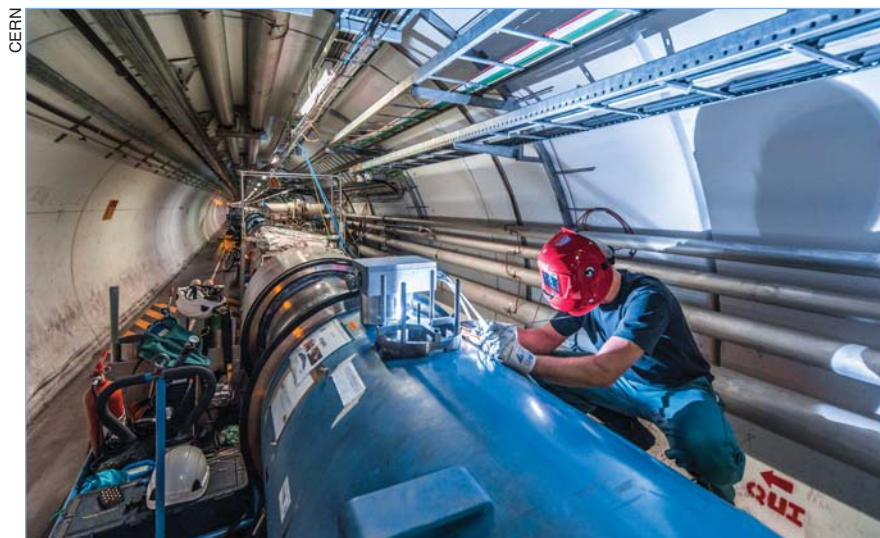
One of the key repairs to the Large Hadron Collider was the welding of more than 27 000 shunts on the 10 000 connections between magnets to provide an alternative path for the high current in case circuit elements lose their superconductivity.
