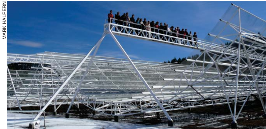
This pair of radio antennas is the warm-up for the Canadian Hydrogen Intensity Mapping Experiment. CHIME team members have climbed up to a platform at the focal line of one of the reflectors.
