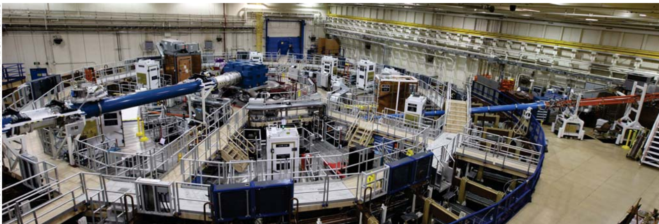
When energy slams a target at the center of the Z pulsed-power machine, the resulting x rays and plasmas are used to study materials, fusion, and astrophysics. The blue tube (left) carries the laser beam that is used for preheating plasmas and for radiographic imaging. X-ray power and energy diagnostics are placed at the far end of the blue and orange pipe (right).
