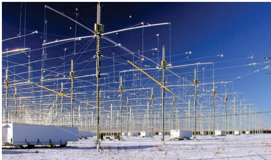
The High Frequency Active Auroral Research Program in Alaska is the world's leading ionospheric heater; with it, the ionosphere can become a plasma-physics laboratory.
