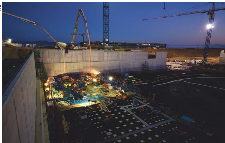
Concrete pouring for the basement of the tokamak complex at ITER began in mid December. Fourteen more pour days will be required over six months to complete the 1.5-meter-thick slab that will support the weight of the tokamak, diagnostic, and tritium buildings.
