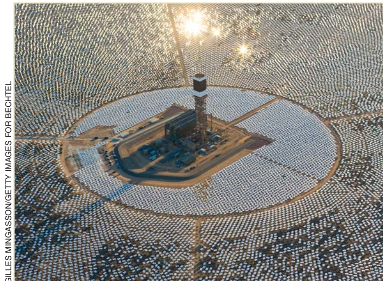
Figure 2. The Ivanpah Solar Electric Generating System, located in California's Mojave Desert, began commercial operation in 2013. The facility uses more than 300 000 tracking mirrors called heliostats to focus sunlight onto boilers atop three towers. The focused sunlight heats water in the boilers to generate steam, which in turn drives conventional turbines. The 377-MW-capacity plant was built with the help of a $1.6 billion loan guarantee from the US Department of Energy.
