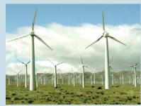
Primarily arising in aerodynamic boundary layers along the rotating turbine blades, the sounds are amplitude modulated, with a characteristic "swish" at a frequency of about 1 Hz. Periodic sounds are more readily per-
