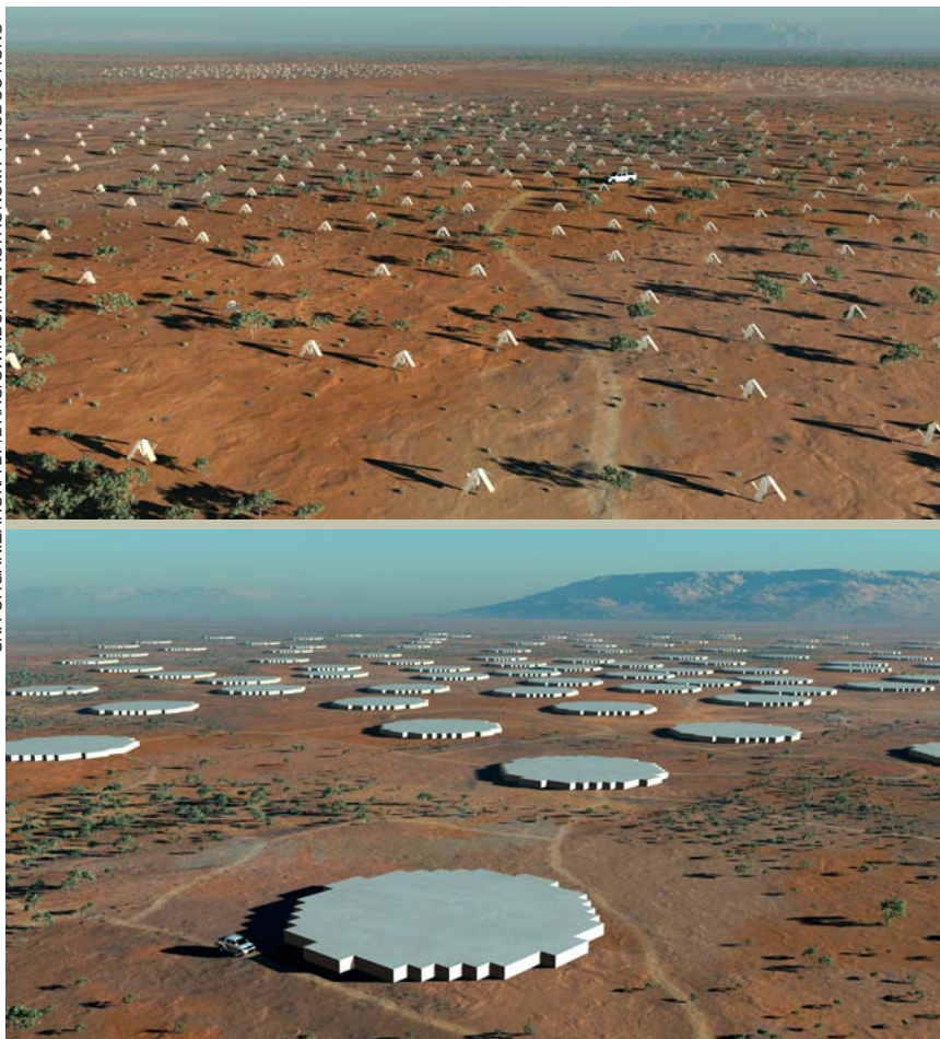
Aperture arrays for low (top) and middle (bottom) frequencies, to be located in Australia and South Africa, respectively, will be part of the Square Kilometre Array.
