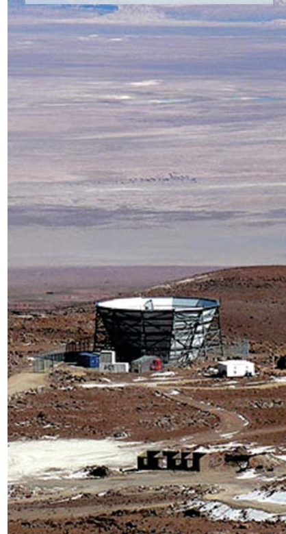
Figure 1. The Atacama Cosmology Telescope, funded by NSF, is a 6-m telescope in the Atacama Desert in Chile. Its remote location and high altitude (more than 5000 m above sea level) minimize atmospheric interference and allow it to collect high-resolution data on the cosmic microwave background.
