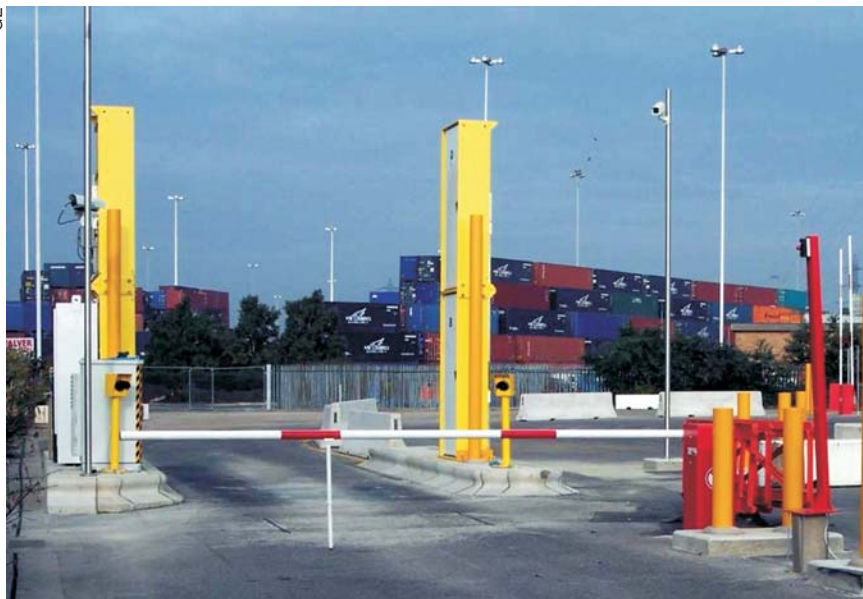
Using tubes lined with boron-10, GE and SAIC have developed a plug-in replacement for the helium-3 neutron detectors in radiation portal monitors, used to scan cargo entering the US for the presence of nuclear materials. Portal monitors, which use large amounts of ^3\text{He} , were blamed for creating a worldwide shortage of the gas.
