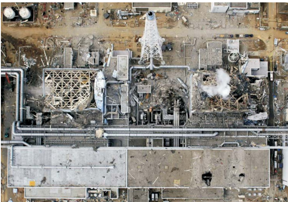
A photo taken from a small, unmanned airplane on 20 March shows damage to the reactors at the Fukushima Daiichi powerplant in the wake of the 11 March earthquake and tsunami.
