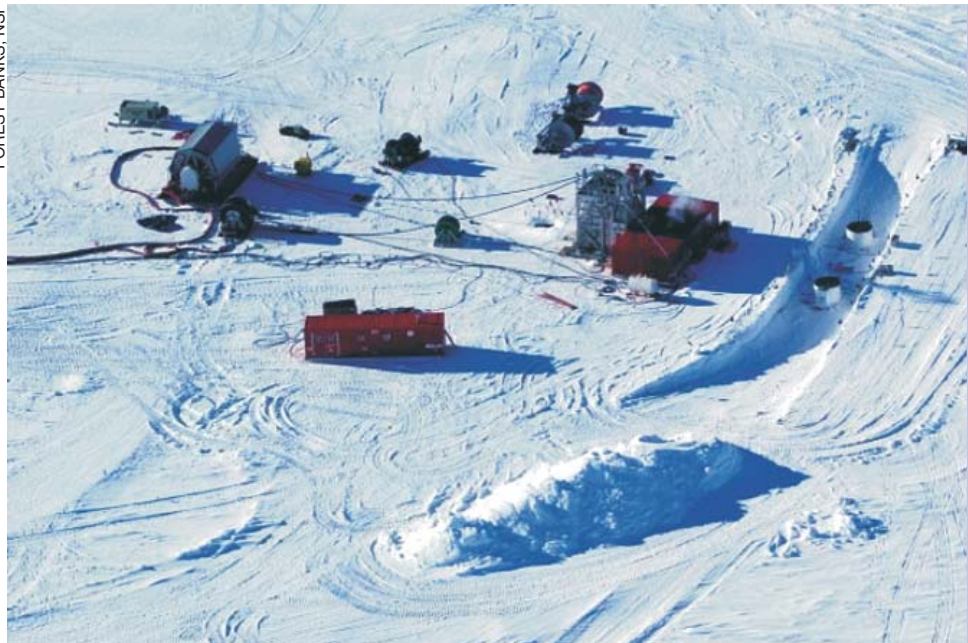
Figure 4. Construction of the IceCube neutrino telescope at the Amundsen-Scott South Pole Station. 9 Under the tallish building right of center, one of the telescope's 80 holes is being drilled to a depth of 2.5 km with hot water coming from a heating plant off left through the red hose to the large cylindrical spool, which unreels hose as the drilling proceeds. Before the water freezes, a kilometer-long string of 60 phototube modules is lowered almost to the bottom to freeze in place. The trench at right holds two tanks of the Ice-Top surface array of ice-Cherenkov detectors that will record charged particles from cosmic-ray air showers.
