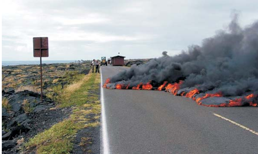
Figure 1. On 13 February 2003, flowing lava from the Pu'u 'O'o volcanic cone inundated Chain of Craters Road in Hawaii Volcanoes National Park on Hawaii's big island. Mobile structures maintained by the park were towed up the road and saved. (Courtesy of the US Geological Survey.)
