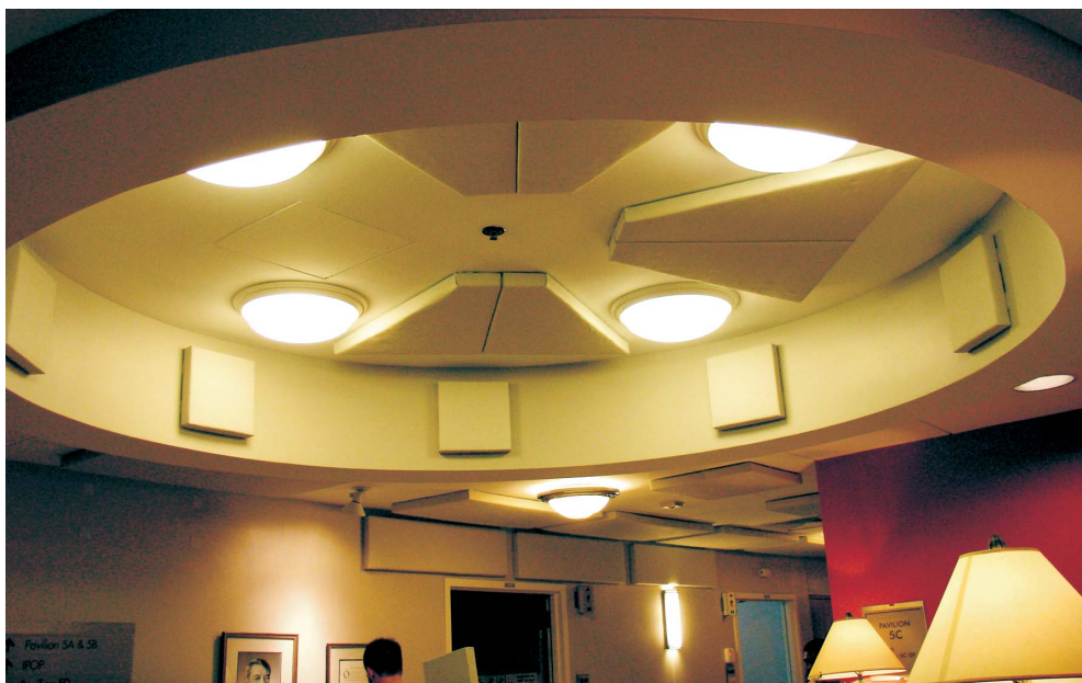
Figure 2. The nurses station in the Weinberg 5C cancer unit of the Johns Hopkins Hospital features a domed circular ceiling. Despite its visual charm, the dome worsens the noise levels. The installed panels reduced the sound level and reverberation time. (Adapted from ref. 1.)
