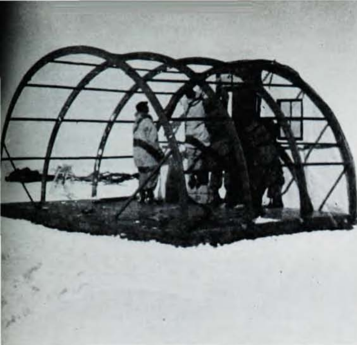
Erecting a prefabricated hut. The floors and framework are of wood and the covering is insulated canvas. Less than a day was needed to build the hut, which is extremely durable.
