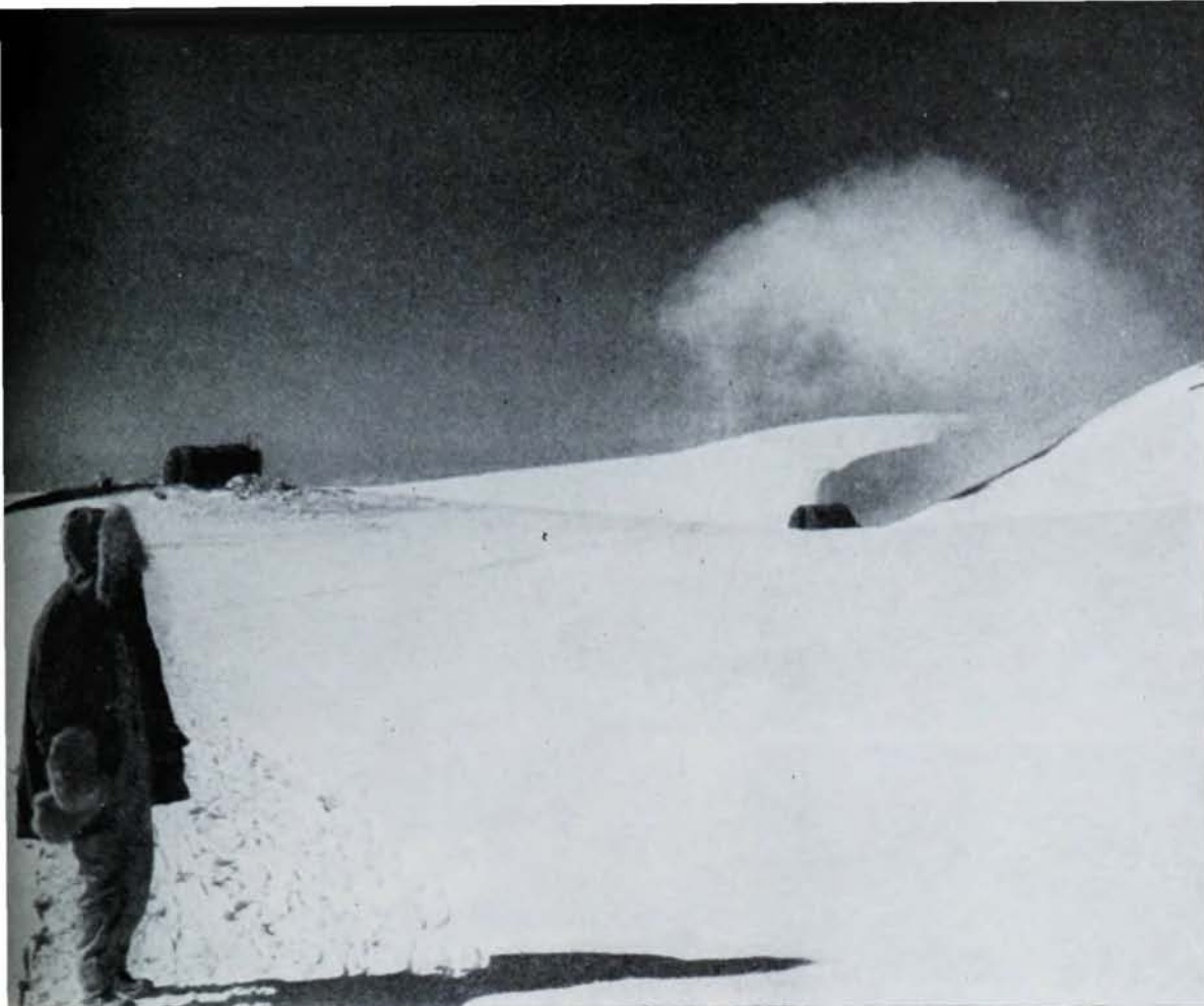
The completed laboratory, with the active crater at the right. The crater is actually over a half-mile away and proved quite docile. The upper hut is 16 x 16 feet in size and contains living quarters for six as well as space for some apparatus. The lower hut, fifty yards away, is occupied by generators and additional equipment. The ridge on which the huts are located is kept permanently free of snow by volcanic steam from the interior of the mountain.
