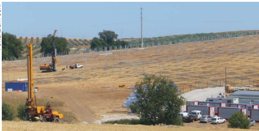
Construction is under way on a 52 000-module solar power plant on a 150-acre hillside in Serpa, southeast Portugal. When the plant is completed in January 2007, it will be among the largest in the world.
