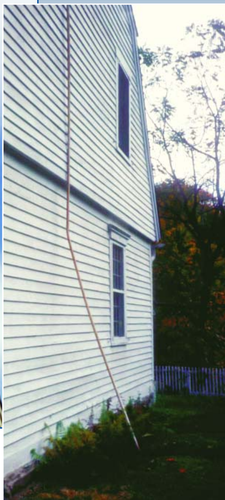
Figure 5. An 18th-century house with a lightning rod of Franklin's 1762 design. The thick, continuous rod can carry tens of kiloamperes of current to ground without harming the house or its foundation.
