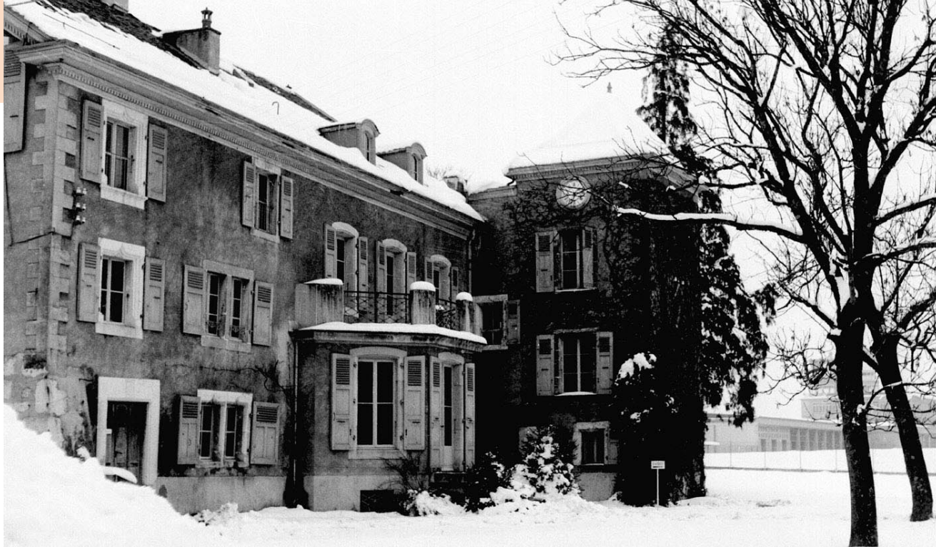
The Villa de Cointrin at the Geneva Airport (whose control tower is visible at right in the background) was CERN's original headquarters. (Courtesy of CERN.)
