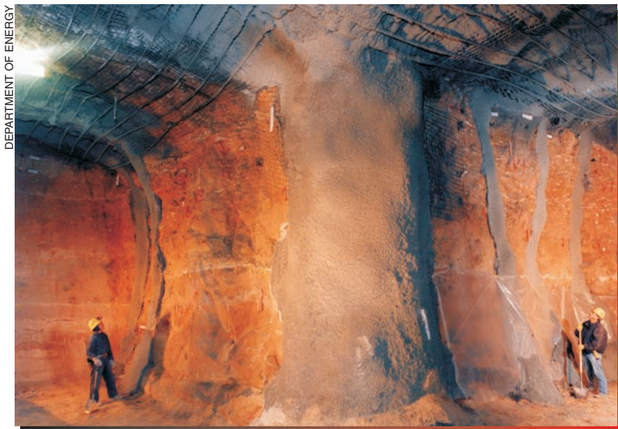
Early tunnel workers at Yucca Mountain are at risk of developing silicosis.
