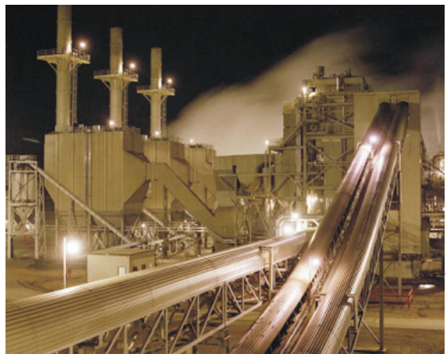
FIGURE 5. BIOMASS POWER PLANT of the Wheelabrator Shasta Energy Co in Anderson, California, delivers 50 MW of electric power. It is fueled by wood from forest residues and lumber-mill wastes from the surrounding area.
