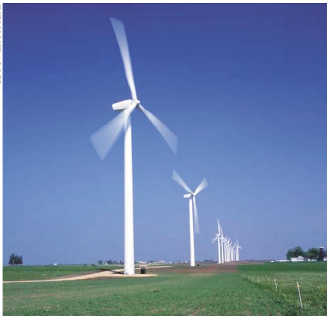
FIGURE 4. MONTFORT WIND FARM in Eden County, Wisconsin. These 20 wind turbines, each with a capacity of 1.5 MW, were put in place last year, replacing an earlier generation. Their 100-ft blades are installed on towers 215-ft high.
