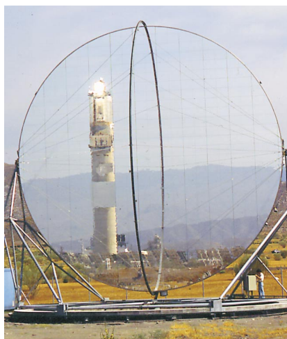
LA PLATAFORMA SOLAR DE ALMERÍA in southern Spain's Tabernas desert is one of two major solar energy research centers in Europe. The reflection in the experimental stretched-membrane heliostat shows one of the center's 84-meter receiving towers.
