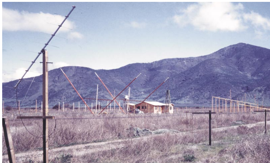
THE RADIO ASTRONOMY OBSERVATORY at Maipú, Chile, in October 1959. In the left foreground is a Yagi radio antenna of the solar interferometer; on the right is the inclined plane of another antenna. In the middle, near the building, the tall V-shaped structures make up the corner reflector. Both the inclined-plane antenna and the corner reflector were used primarily for observations of Jupiter.
