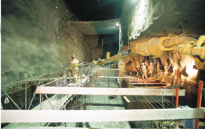
EXCAVATION for the Compact Muon Solenoid experiment contributed to the Large Hadron Collider's cost overrun.
