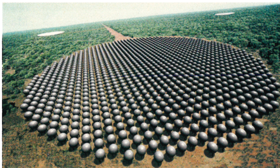
ARRAYS OF SPHERICAL LENSES are what Australian radio astronomers hope will prove economically and technologically best for the Square Kilometre Array. (Computer generated image courtesy of Ben Simons/Sydney VisLab/CSIRO.)
