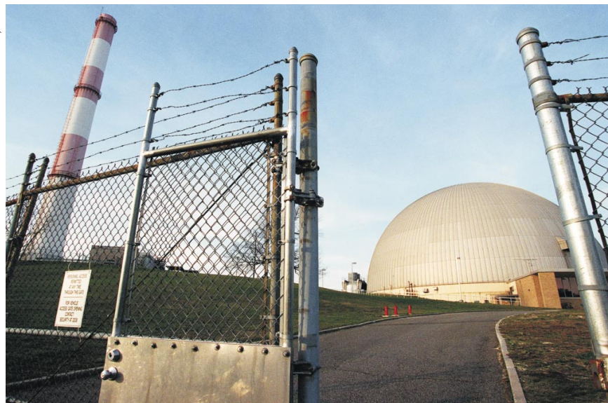
BITTER END: Closing the gate on the HFBR at Brookhaven National Laboratory.
