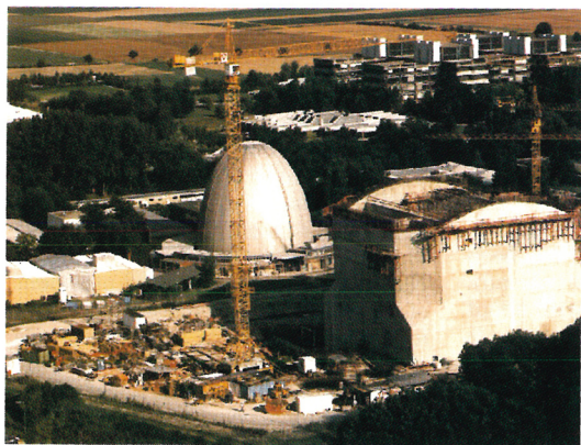
THE CONTROVERSIAL RESEARCH REACTOR FRM2 (for Forschungsreaktor München 2) is being built next to its predecessor, the Atomei (atom egg) in Garching, north of Munich. This photo was taken last July.
