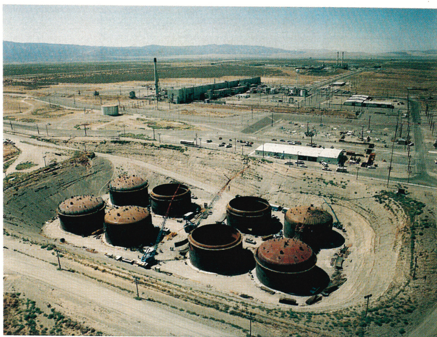
FIGURE 4. DOUBLE-SHELL TANKS under construction at DOE's Hanford site, near Richland, Washington. These tanks, which went into service in 1986, are 22.8 m in diameter and 15.2 m high and have a capacity of about 4.4 million liters each. Each was constructed out of two carbon steel shells and was encased in concrete before being buried. Note the riser ports on the tops of the enclosed tanks. The long building with the smokestack in the background is the PUREX (plutonium and uranium extraction) reprocessing facility. (Photo courtesy of DOE Richland Operations Office.)
