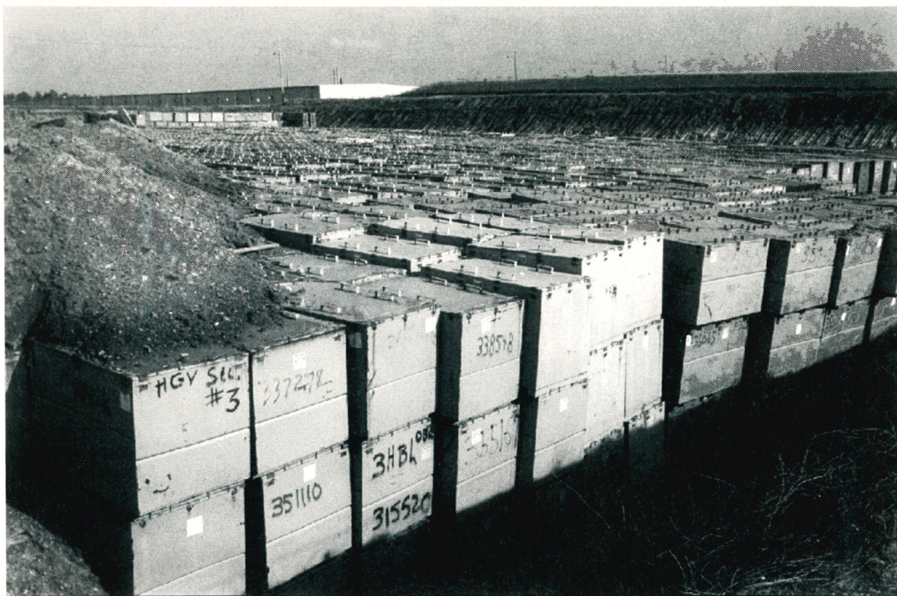
FIGURE 5. LOW-LEVEL WASTE being buried in an engineered trench at the Savannah River site early in 1994. The trench was designed to hold more than 30 000 carbon steel boxes of waste, each measuring 4 by 4 by 6 feet. When this trench was filled in March 1995, the trench burial of waste at the Savannah River Site was stopped. LLW waste there is now being stored in covered structures. (Photo courtesy of DOE.)
