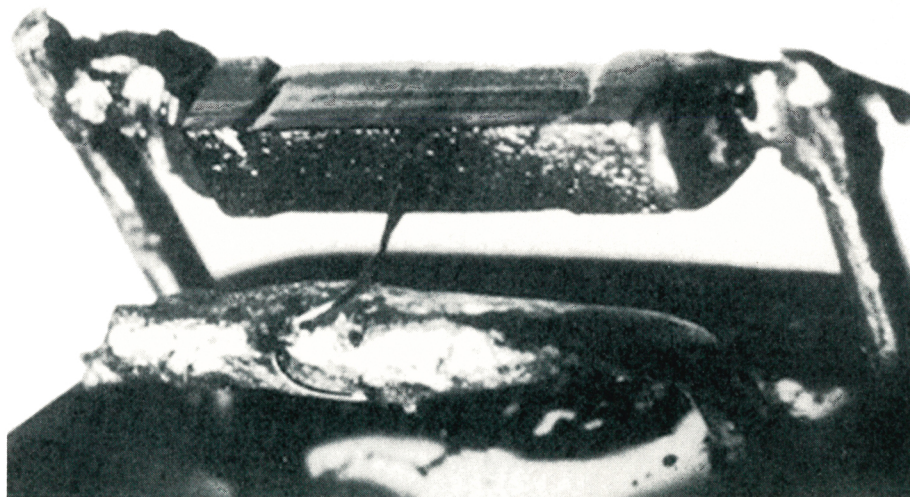
FIGURE 2. FIRST GROWN-JUNCTION TRANSISTOR. Contact was made to the base region by manipulation of a gold wire under a microscope.
