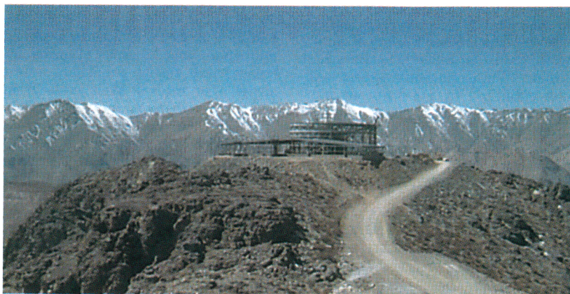
GEMINI SOUTH, under construction on Cerro Pachon, Chile, is scheduled to see first light in 2000, and to be fully operational in 2001.
