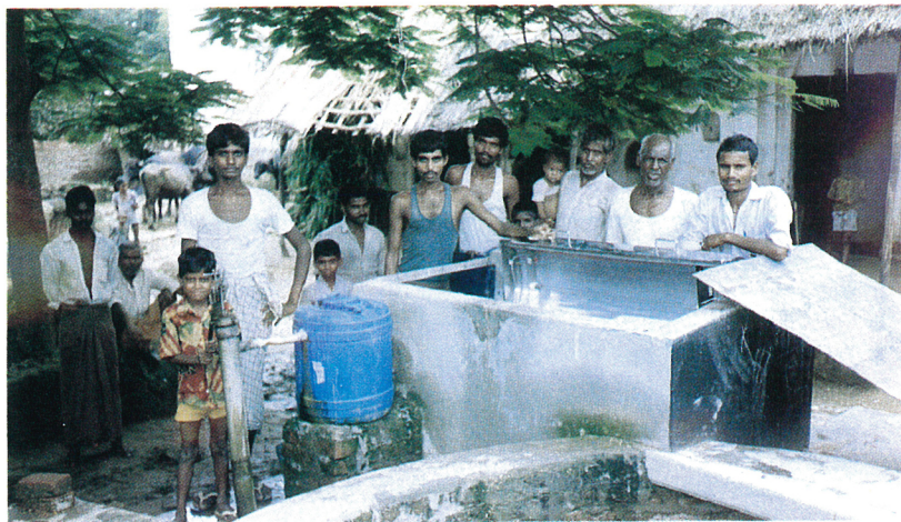
A WATER PURIFICATION UNIT, open for maintenance, surrounded by villagers in Bhupalpur, India. Water is pumped into the blue plastic holding tank and then is disinfected by flowing past the UV lamp in the unit. No women appear in the photo because, although they typically attend to the community's water needs, "it would be culturally inappropriate for them to pose for a male stranger [the photographer]," Ashok Gadgil explains. (Photo courtesy of Urminus Industries.)
