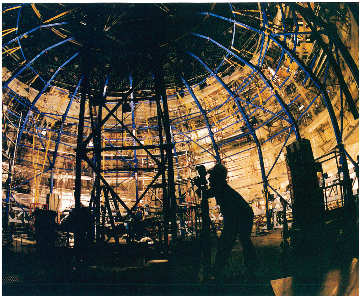
NO DETECTOR'S heavy-water containment vessel in March, as one of its 130 transparent acrylic panels was being led into place. Through the vessel's still open top one can see part of the geodesic array of 9500 photomultiplier tubes that will look for Čerenkov light coming out through the walls of the 12-meter-diameter spherical vessel. When the vessel is completed next year, the dust covers will have come off the phototubes, and everything outside the acrylic vessel, including the phototubes, will be immersed in light water. SNO is 2 kilometers underground in a northern Ontario nickel mine. (Courtesy of Sudbury Neutrino Observatory.) FIGURE 4
